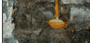
Mushroom on a Foundation Wall
